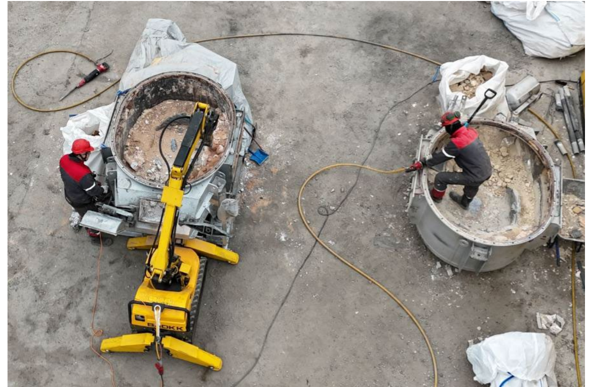
Casting Machine Demolition
