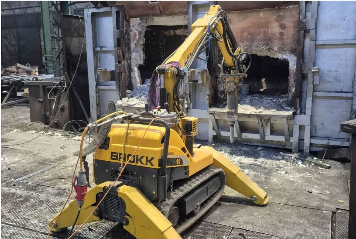
Heat-Treatment Furnace Demolition
