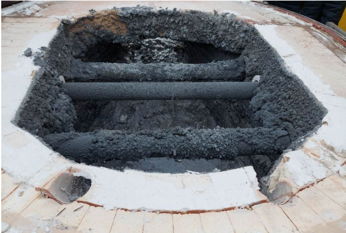
Before the refurbishment
