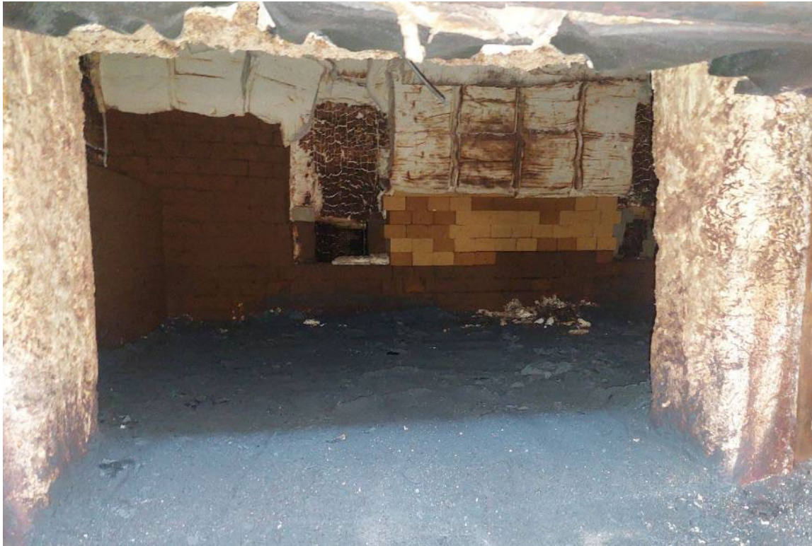
Before the refurbishment
