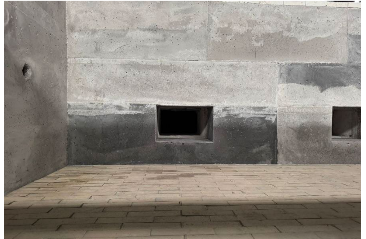
After the refurbishment
