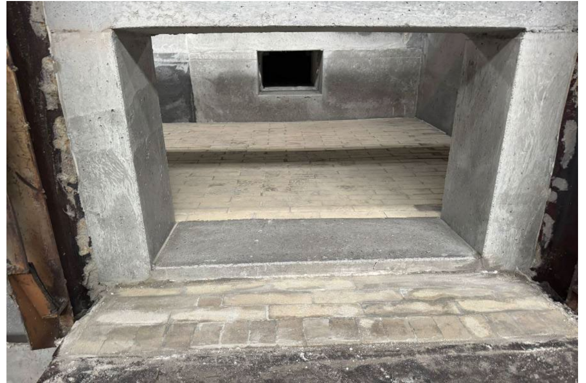
After the refurbishment
