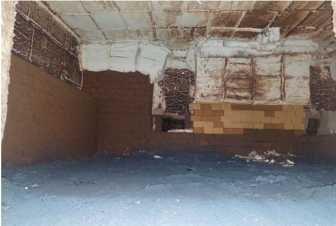
Before the refurbishment
