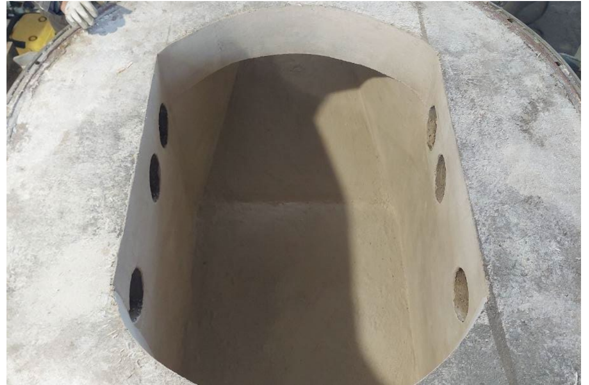
After the refurbishment
