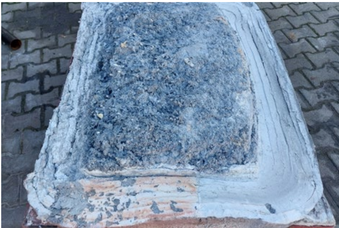
Before the refurbishment
